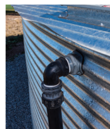
50mm Inlet for Steel Liner Tank
